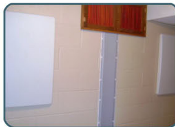
Two wall anchor covers and one well duct window well drain.
