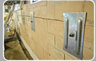
Foundation Supportworks Wall Anchor System Installed
