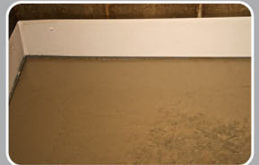
Waterguard system installed
