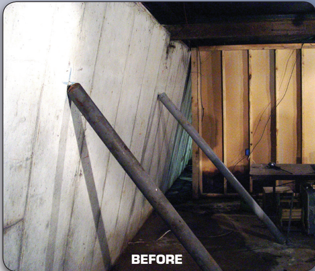
Basement wall severely tipping in at the top.
