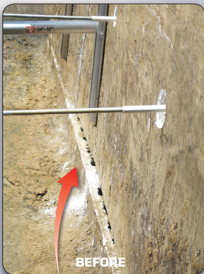
Block wall pushing in several inches at the bottom.
