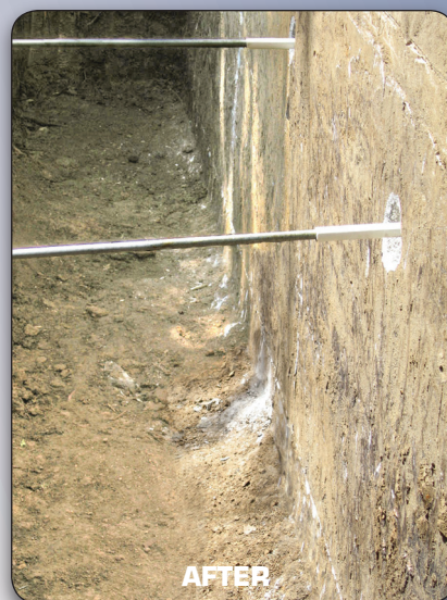
After excavation of soil, the wall is stabilized and returned to a straight position.
