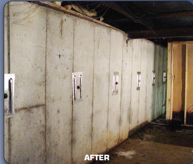
Wall is immediately returned to its original position after soil is removed and Geo-Lock™ Anchors are installed.
