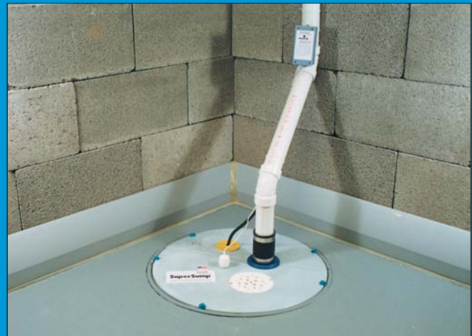
Finished DryTrak® and SuperSump® installation. (over)
