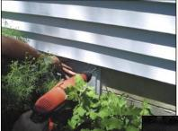
CleanSpace Vent Covers permanently attach to your foundation walls with drilled in anchors - so they will never come off.
