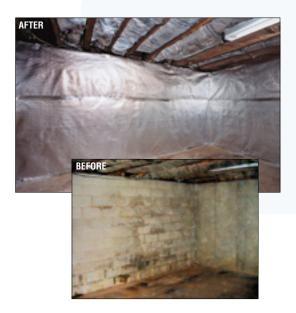
he ThermalDry® Basement Wall System stops water vapor, drains wall leaks, and does something the other three systems cannot do – it reflects up to 97% of the indoor heat back into the basement. This saves energy and money because your heat is not absorbed and lost into the perpetually cold basement walls.
